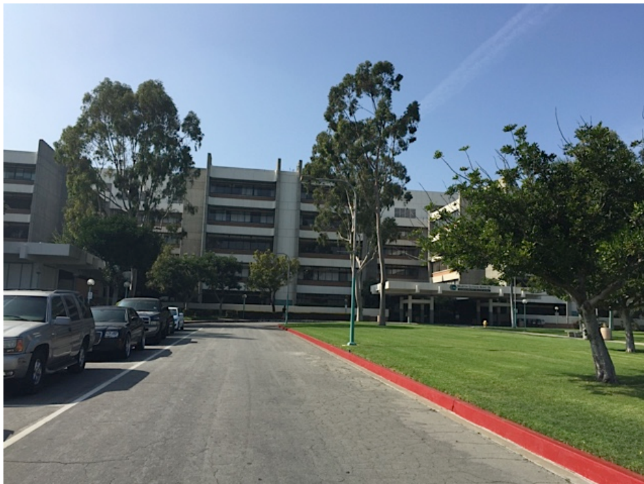
Figure 16 View of Existing MACC from Southern Portion of Main Entry Driveway
