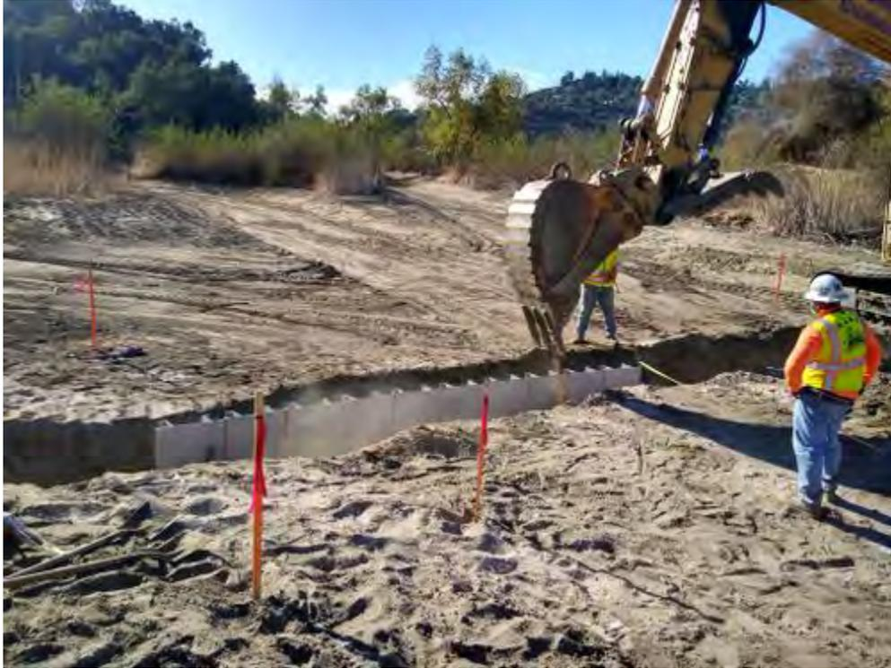
photo\_3-sheet pile install.jpg
