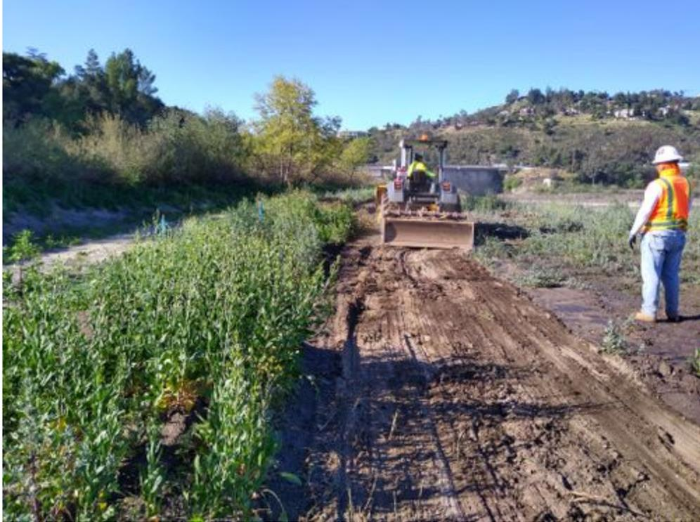
photo\_1-skip loader clearing esa fenceline.jpg
