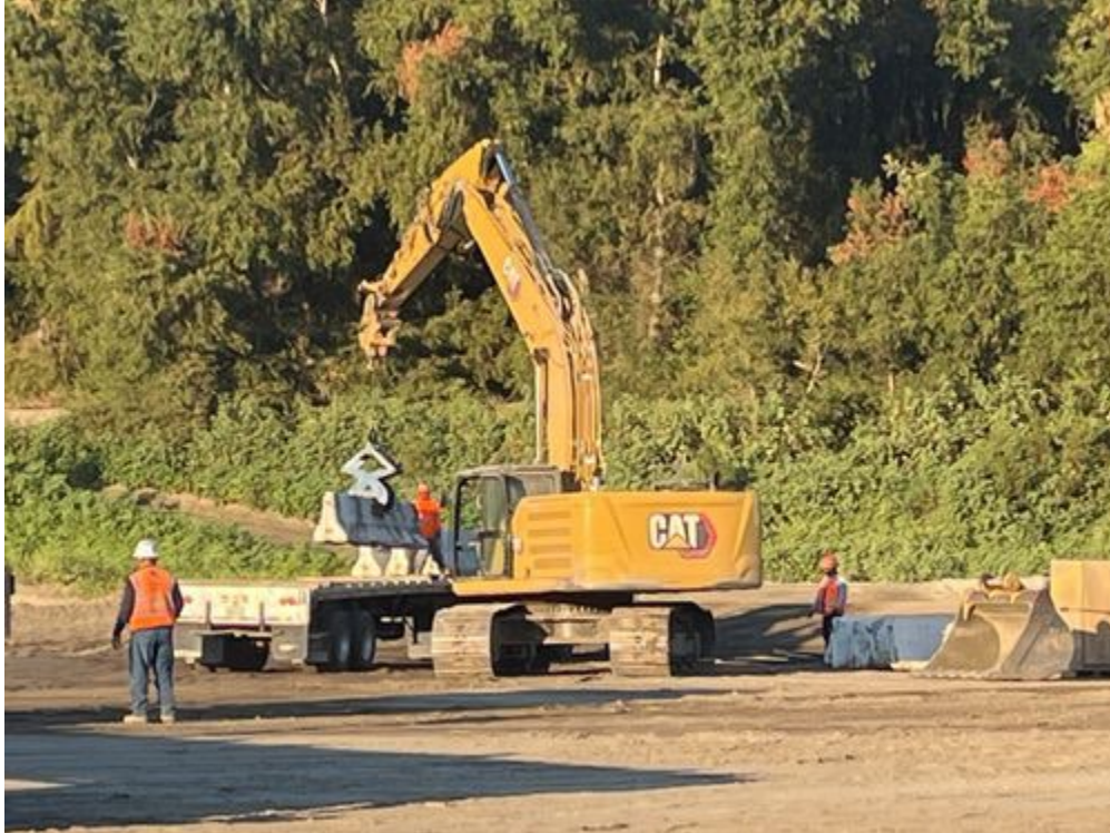
Excavator_load_k-rail_on_truck_faceSW.jpg -118.17550625 34.18809035277778
