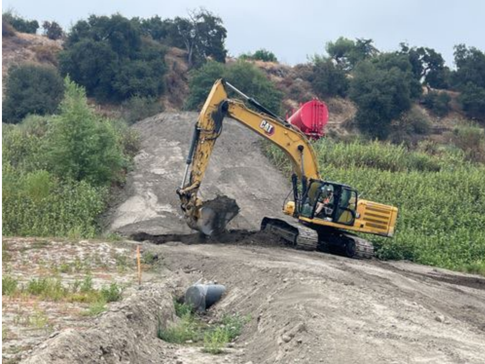
Dig_trench_to_pull_up_drainage_pipe_faceE.jpg -118.17408098888889 34.18718900555555
