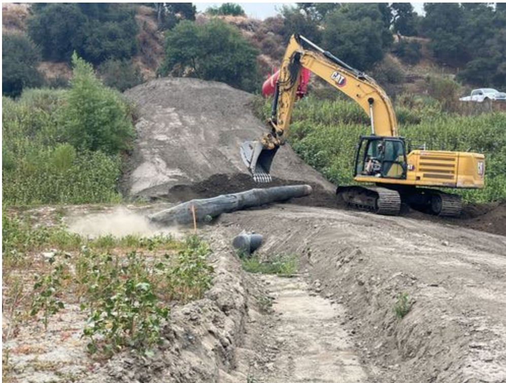
Pull_drainage_pipe_from_access_road_faceE.jpg -118.17410094444445 34.18722446111111
