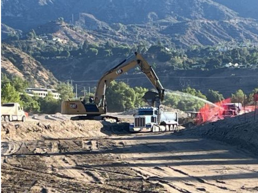
Excavator_filling_dumptruck_with_sediment_facingN.jpg -118.17292020555556 34.191040916666665
