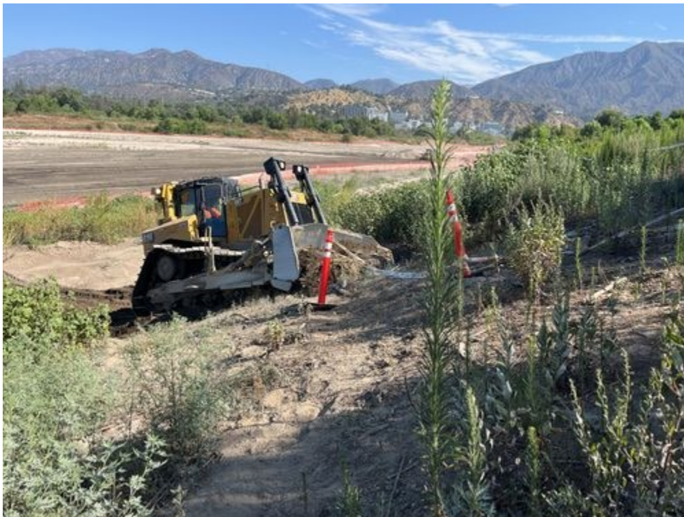
Filling_erosion_with_sediment_faceNW.jpg -118.17326695277778 34.18816162222222
