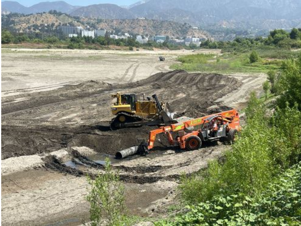
photo_4-low_flow_crossing_installation_facingNW.jpg -118.17444023611111 34.185940563888884
