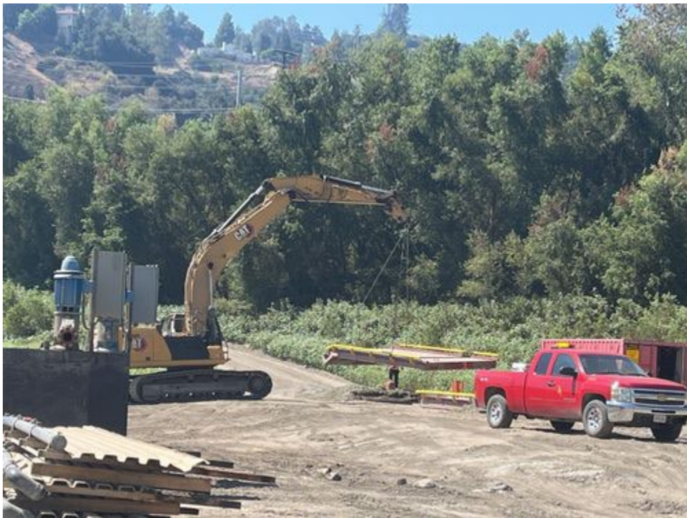
Excavator_remove_weigh_station_plate_faceSW.jpg -118.17608258333334 34.18824507222216
