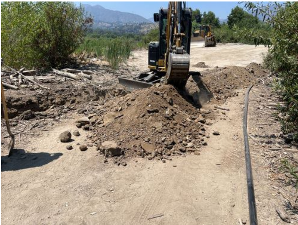
photo_3-burying_water_pipe_facingN.jpg -118.17312034444446 34.18733314999999
