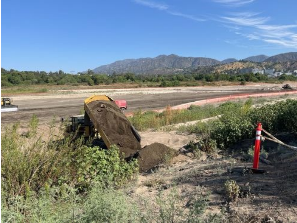
Deposit_sediment_for_erosion_backfill_FaceNW.jpg -118.17330282222223 34.18817428888889
