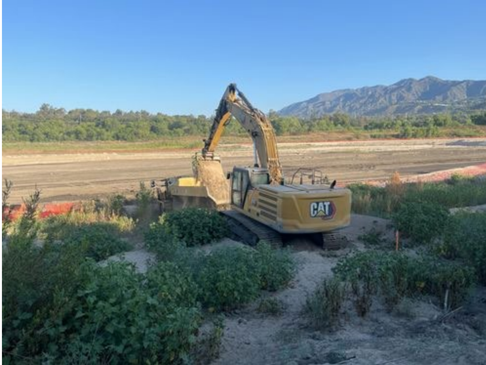
Remove_sand_sediment_below_erosion_area_faceNW.jpg -118.17325286111111 34.188231797222215
