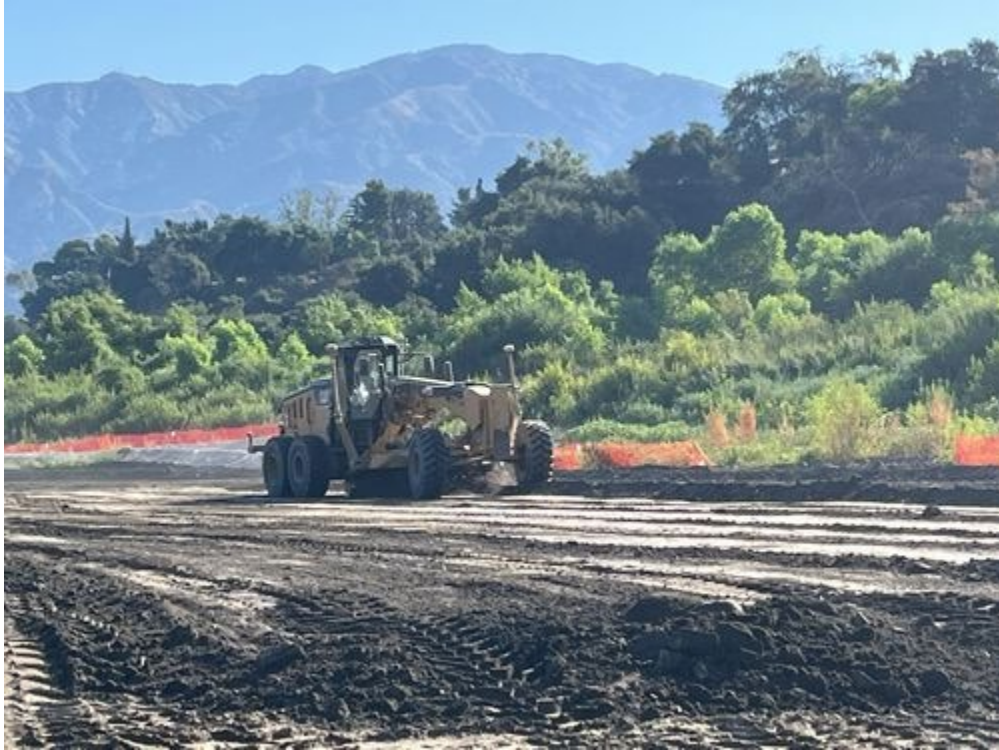
Grading_roads_for_truck_access_facingNE.jpg -118.175189 34.18812011111111
