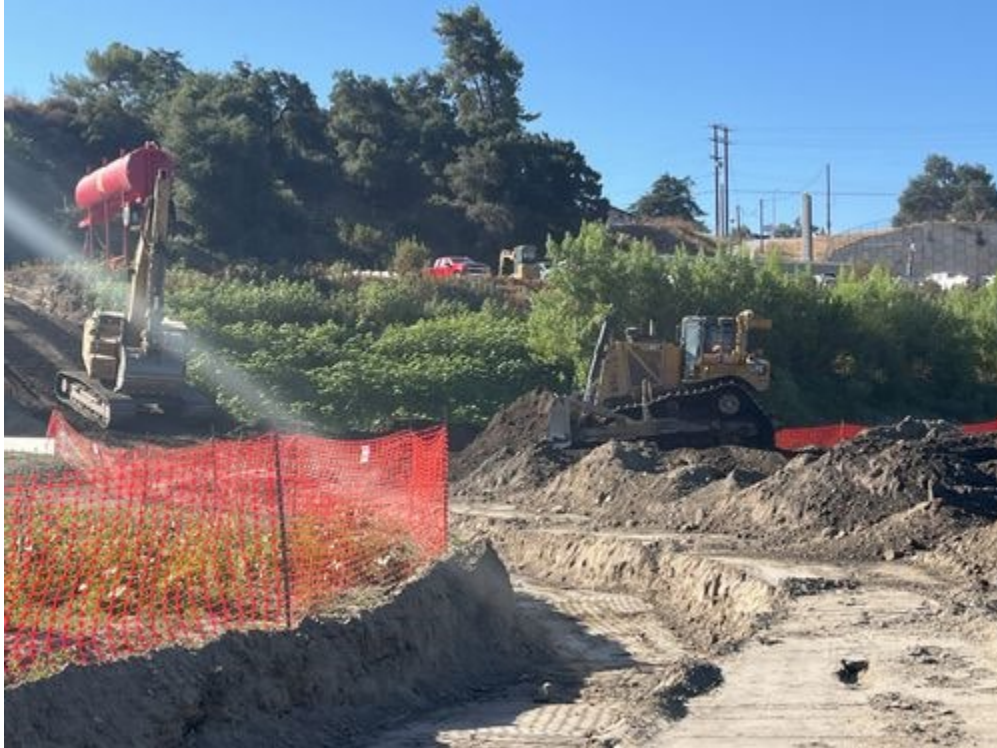
Backfilling_over_drainage_pipe_faceSE.jpg -118.17409591666667 34.18733065555555
