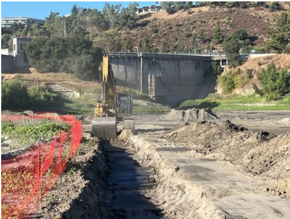
Excavator_digging_drainage_trench_faceS.jpg -118.17389746388889 34.187810049999996
