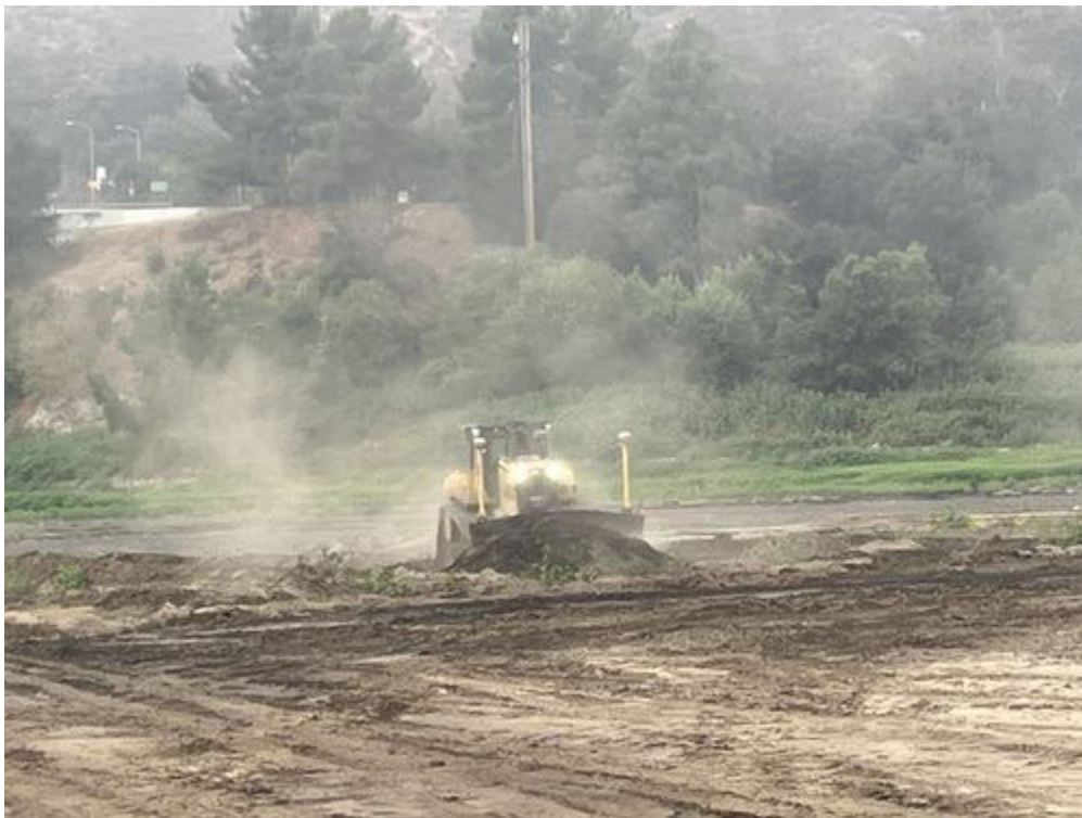
bulldozer_distribute_sediment_facingSW.jpg -118.17391494444445 34.188267463888884
