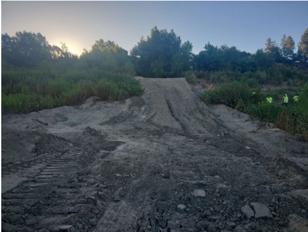
SideSlope_erosion_filled_in_facing_E.jpg -118.1734402222223 34.18831238055555
