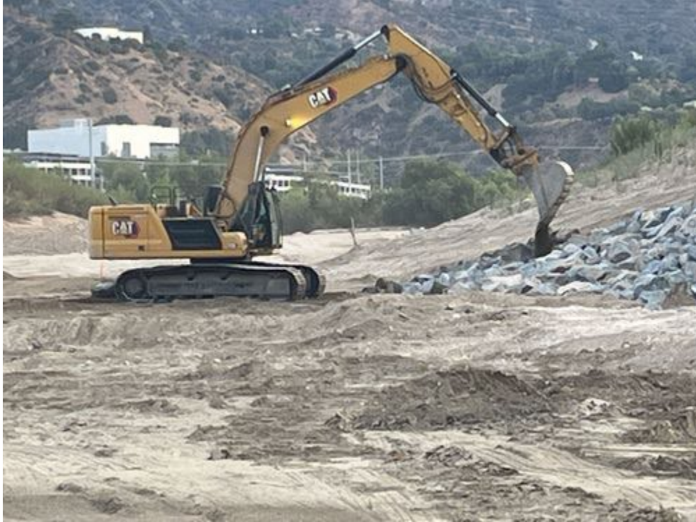
Excavator_adding_rip_rap_east_side_facingN.jpg -118.17309068611111 34.19041440555555
