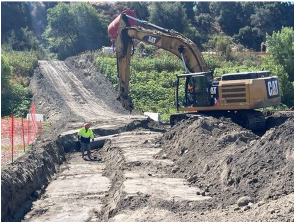
Installing_drainage_pipe_faceSE.jpg -118.17415041666668 34.18716109444444
