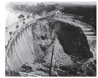
This sediment has built up behind the dam, threatening to block the stormwater release valves that allow dam operators to release water down the Arroyo Seco in a controlled fashion.
