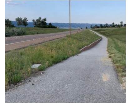
4) Side Path along Interstate
