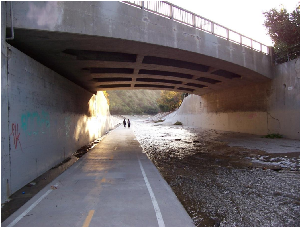
Section 1350 Looking Downstream
