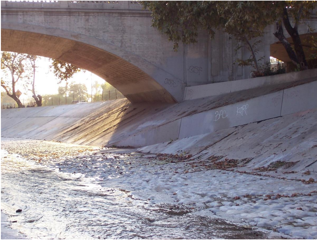
Section 1520 Looking Downstream Right Bank Bridge Abutment
