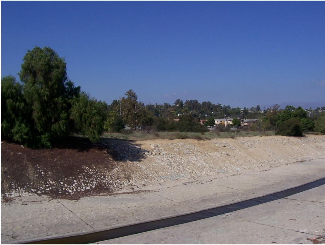
Section 2191.66 Looking Upstream Right Bank
