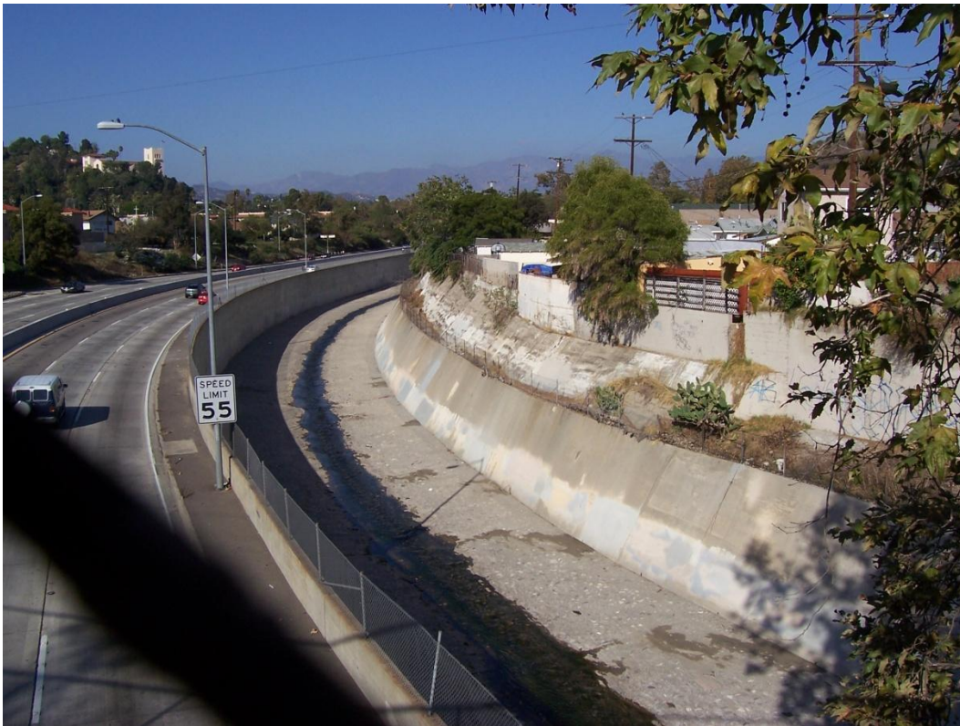
Section 508 Looking Upstream Right Bank
