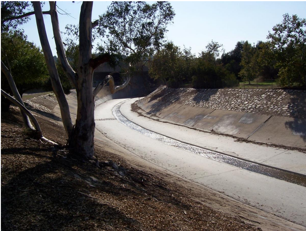
Section 2383 Looking Downstream
