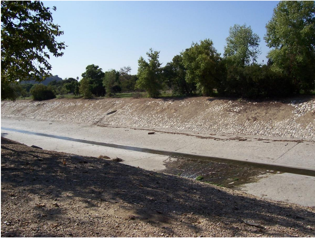
Section 2212.30 Looking Downstream Right Bank
