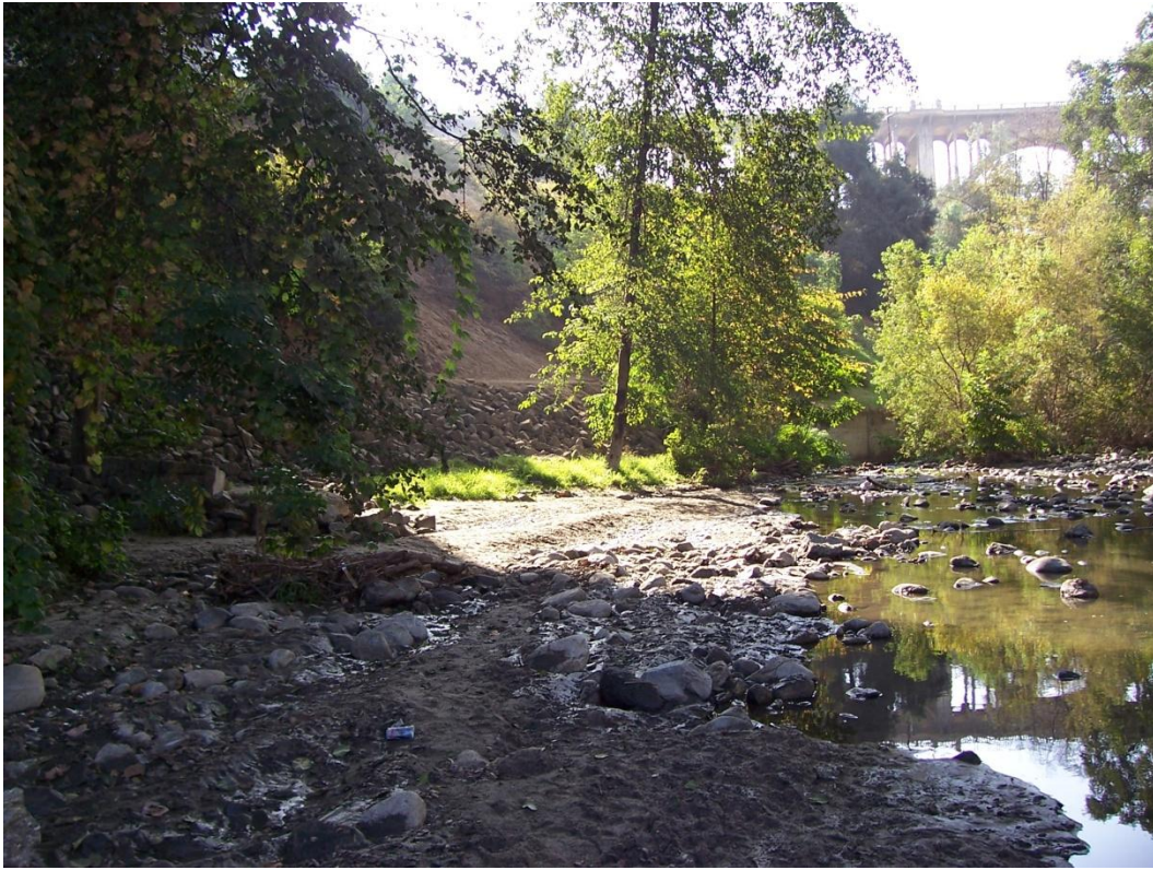
Section 2795 Looking Downstream Left Bank
