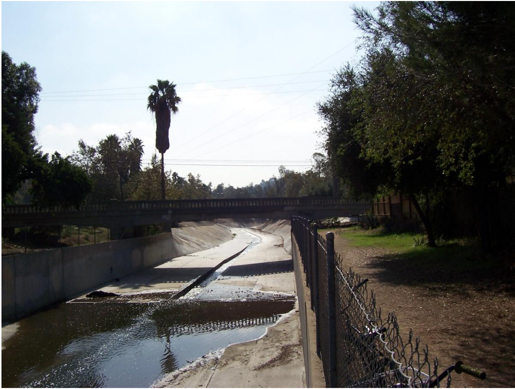
Section 2475 Looking Downstream
