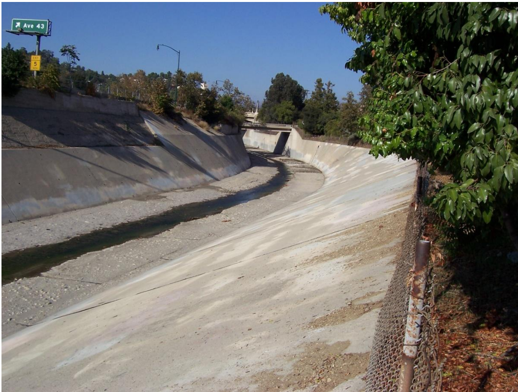
Section 405 Looking Upstream
