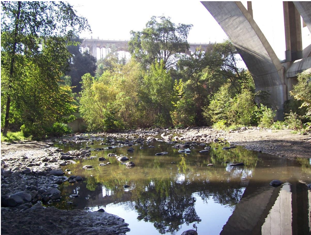
Section 2795 Looking Downstream
