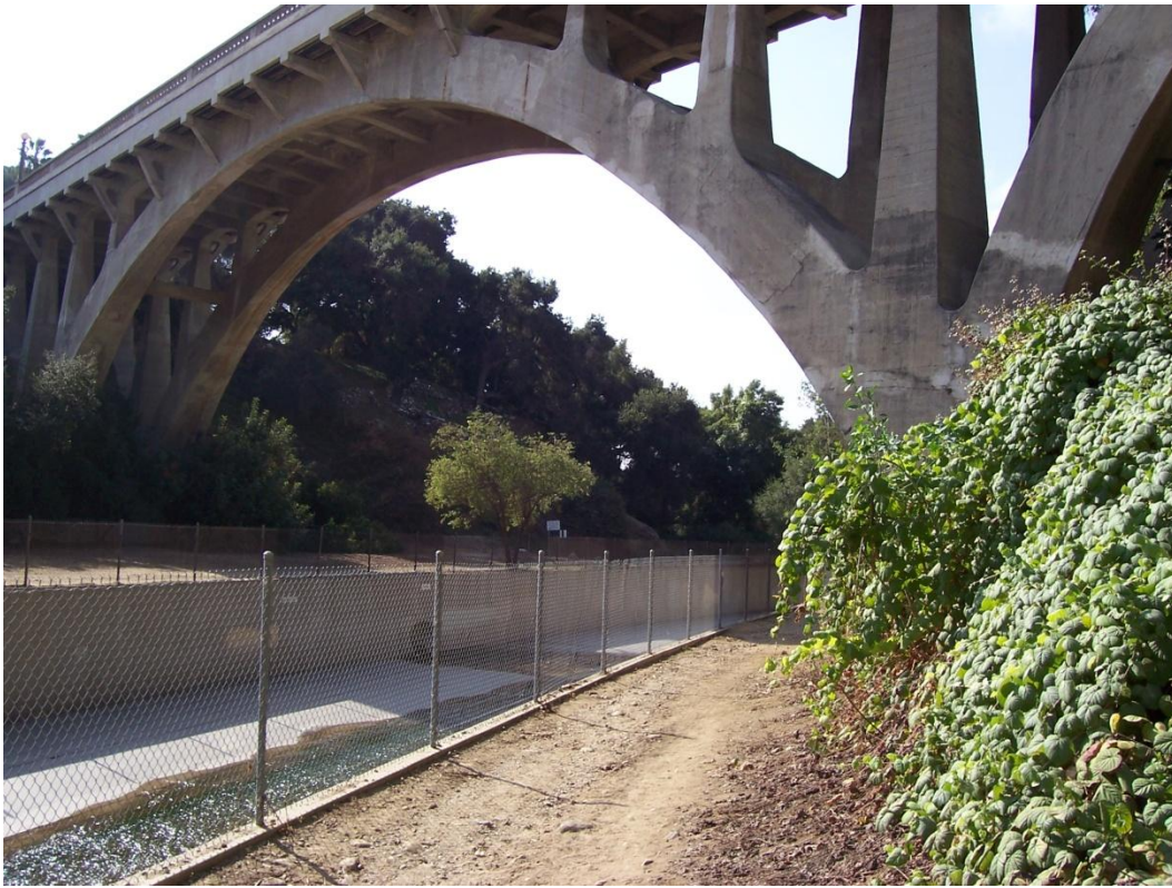
Section 2560 Looking Downstream
