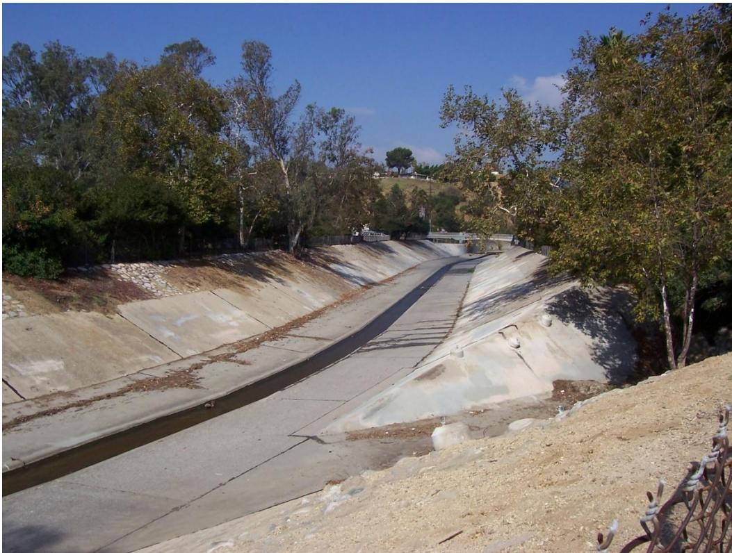
Section 2380 Looking Upstream
