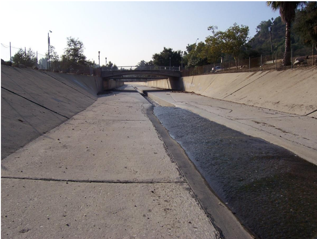
Section 2930 Looking Downstream
