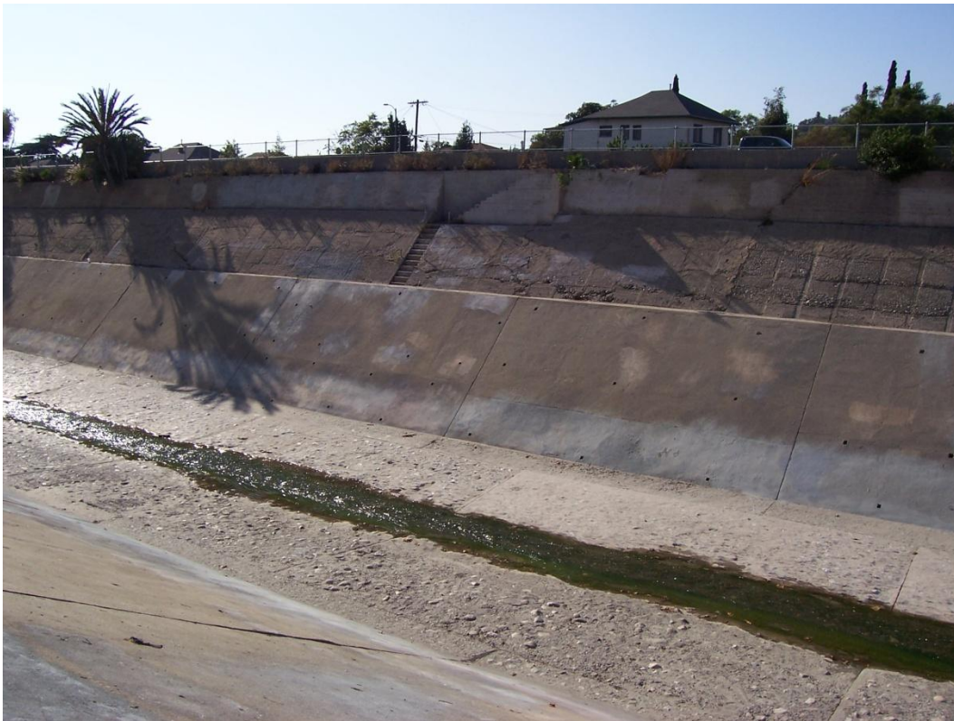
Section 405 Looking Downstream, Stairs
