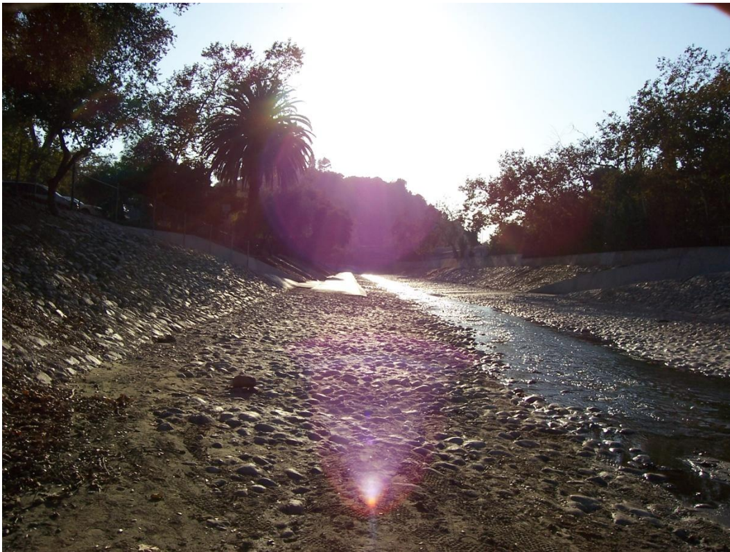
Section 1930 Looking Downstream
