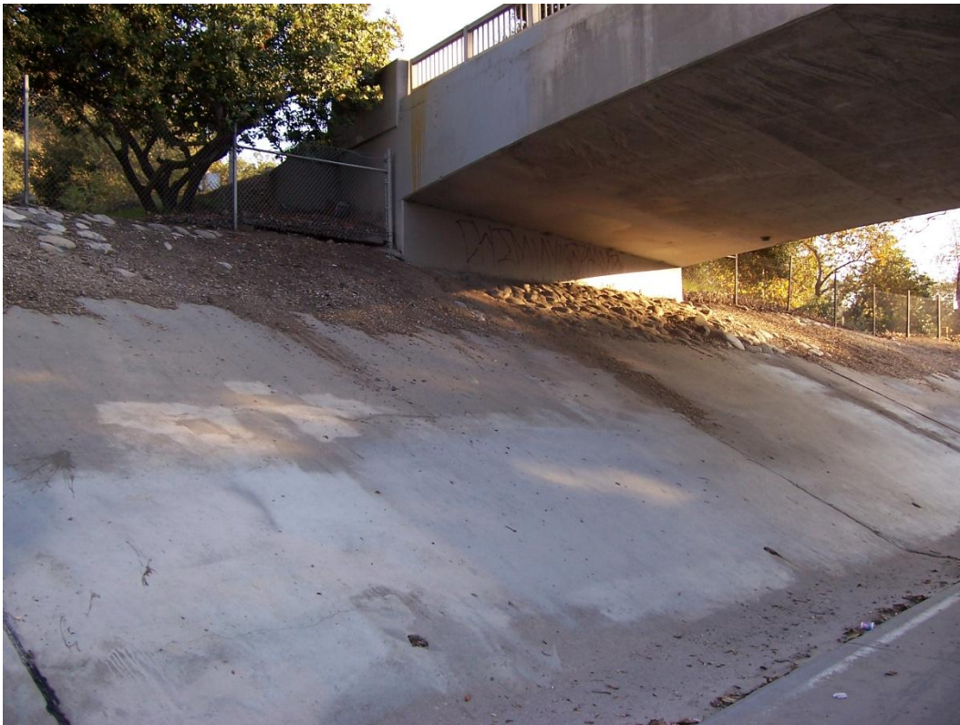
Section 1535 Looking Downstream Left Bank Bridge Abutment
