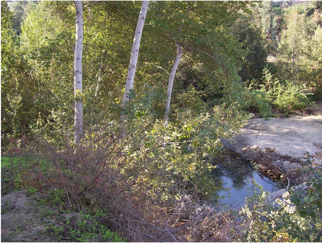
Section 2820 Looking Downstream of Cutoff
