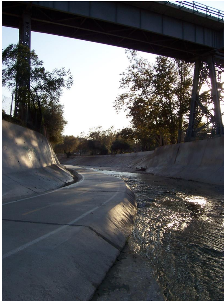
Section 1700 Looking Downstream
