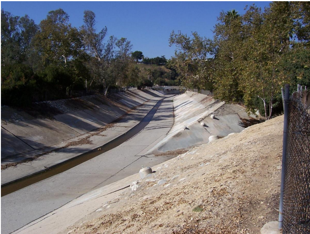
Section 2383 Looking Upstream
