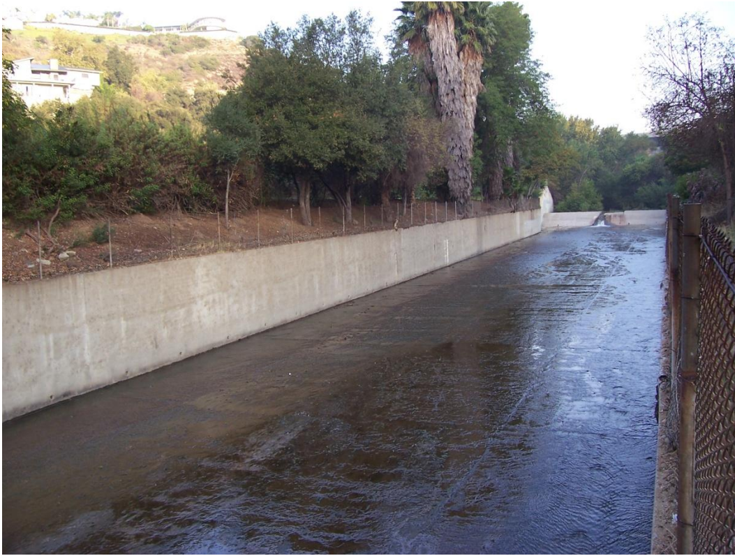
Section 3090 Looking Upstream
