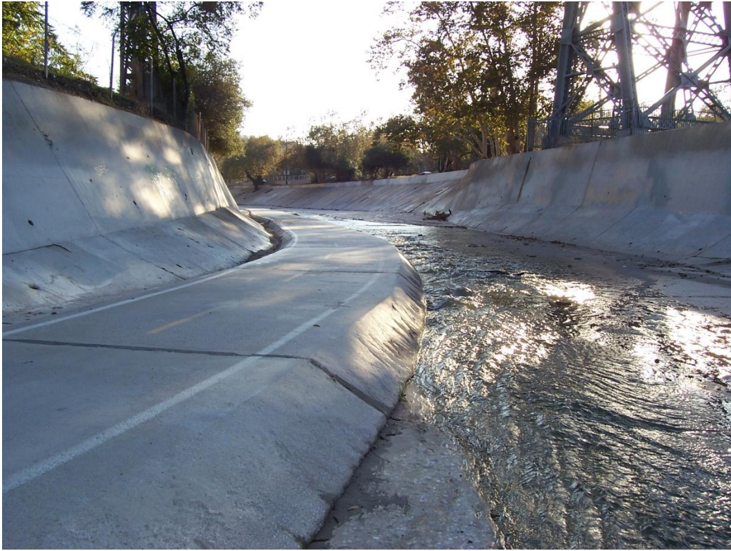
Section 1700 Looking Downstream Past Bridge
