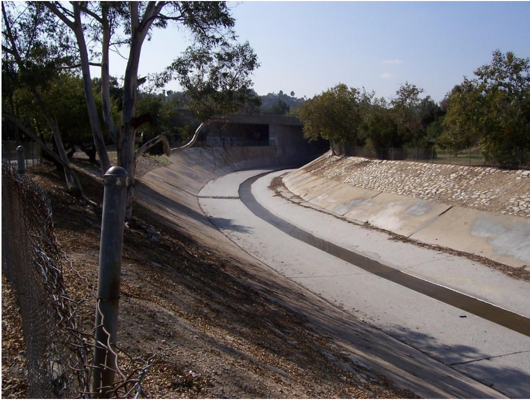
Section 2380 Looking Downstream
