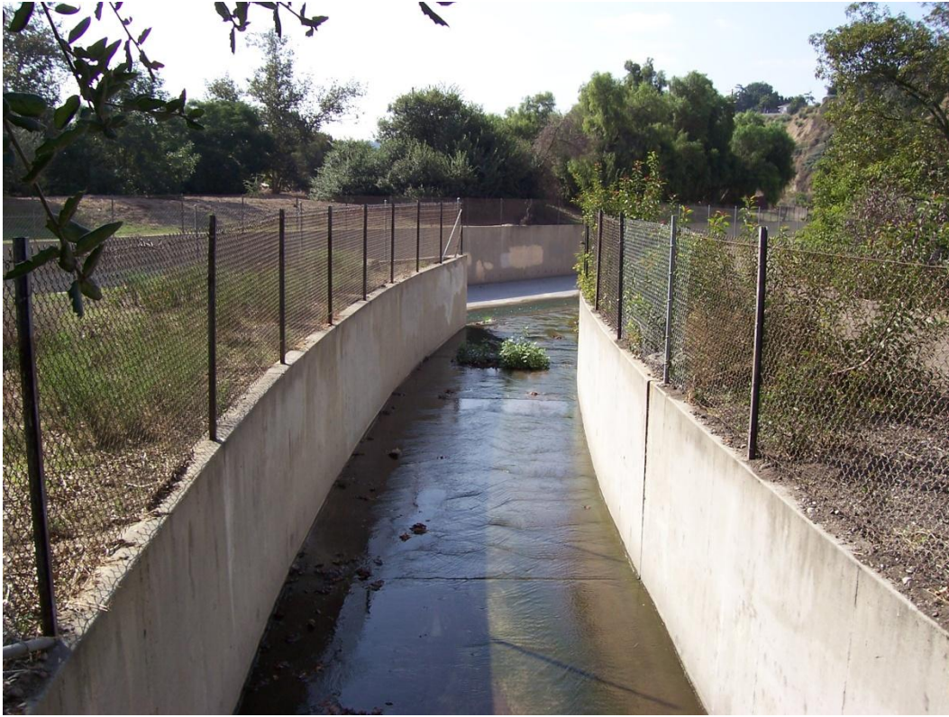
Section 2530 Looking Downstream Lateral Right
