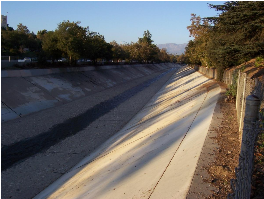
Section 598 Looking Upstream
