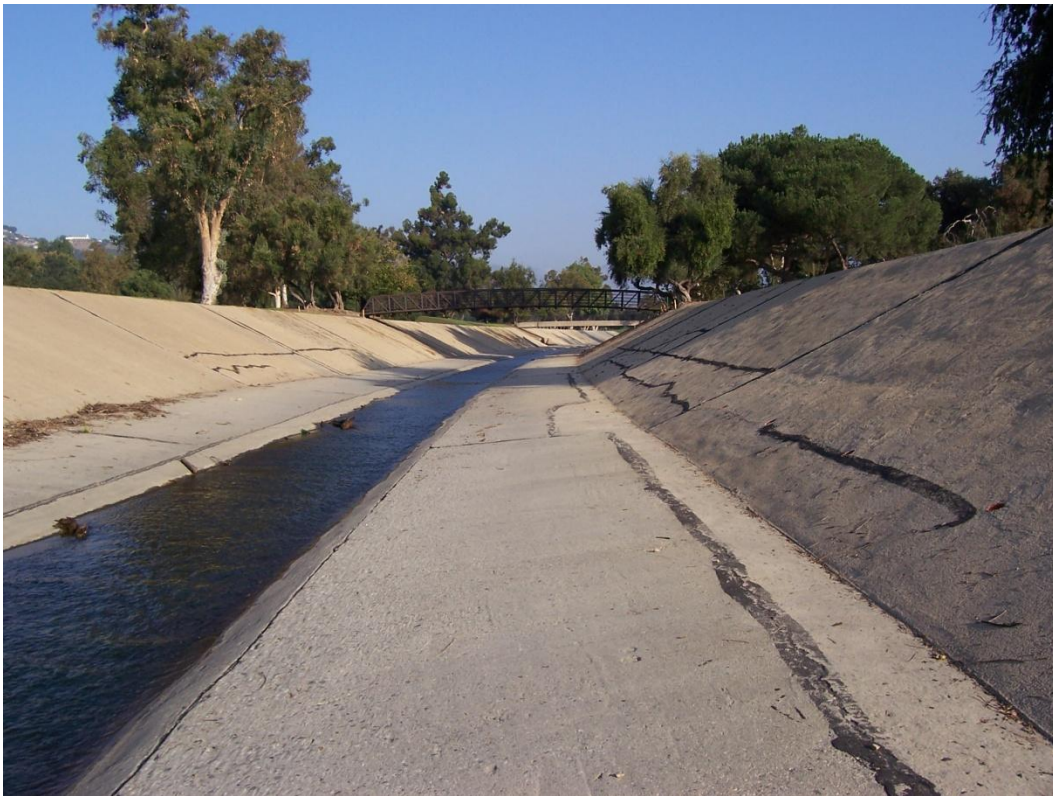
Section 3001.36 Looking Upstream
