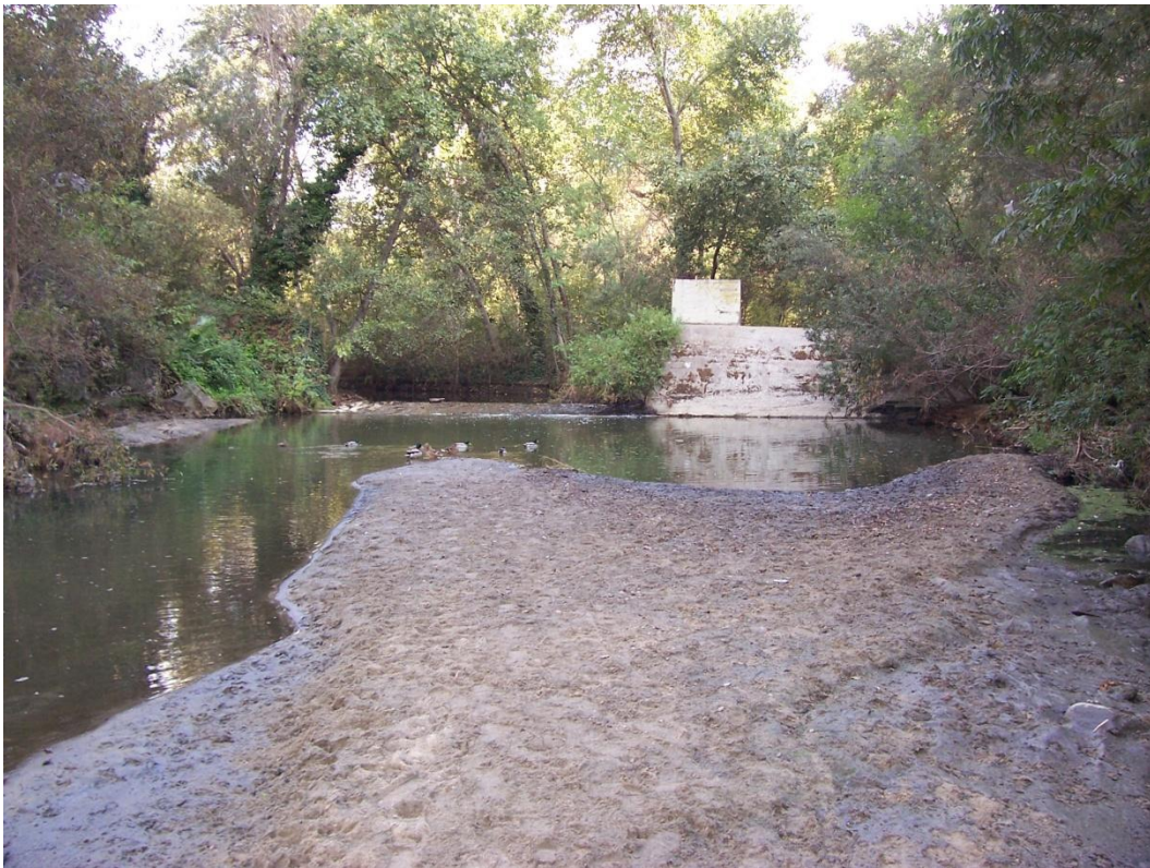
Section 2795 Looking Upstream
