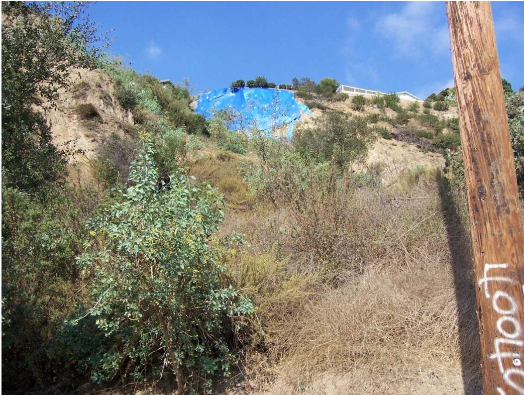
Section 2509 Right Bank Mudslide
