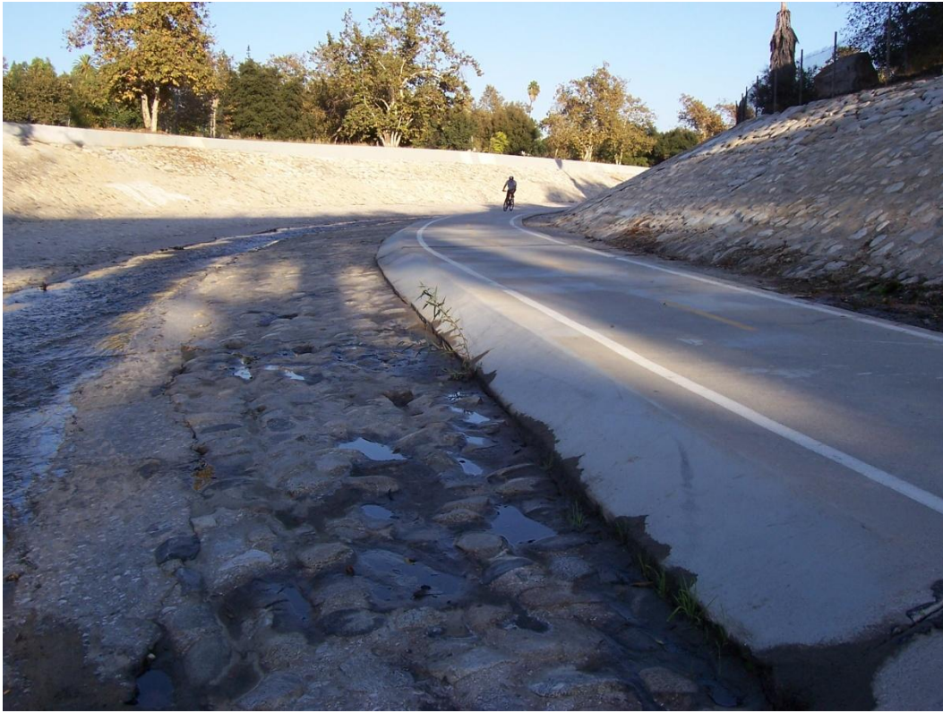
Section 1700 Looking Upstream
