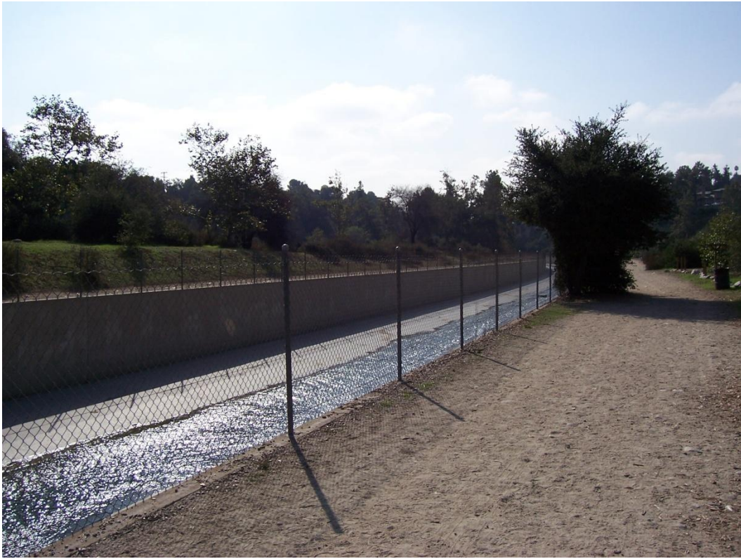
Section 2655 Looking Downstream Left Bank
