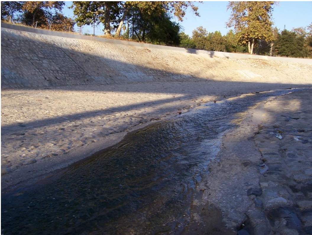
Section 1700 Looking Upstream Right Bank
