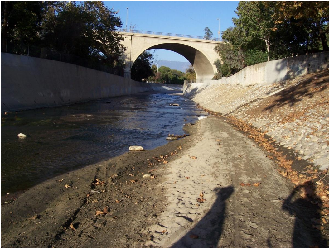
Section 1930 Looking Upstream
