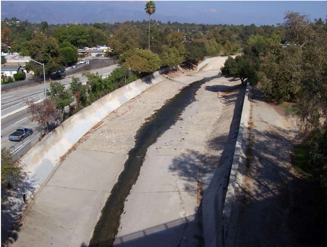
Section 1995 Looking Upstream
