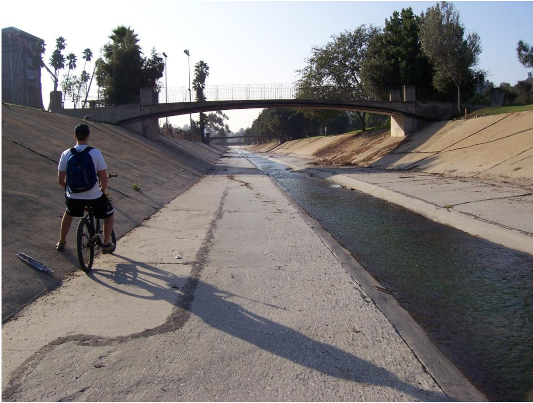
Section 3001.36 Looking Downstream
