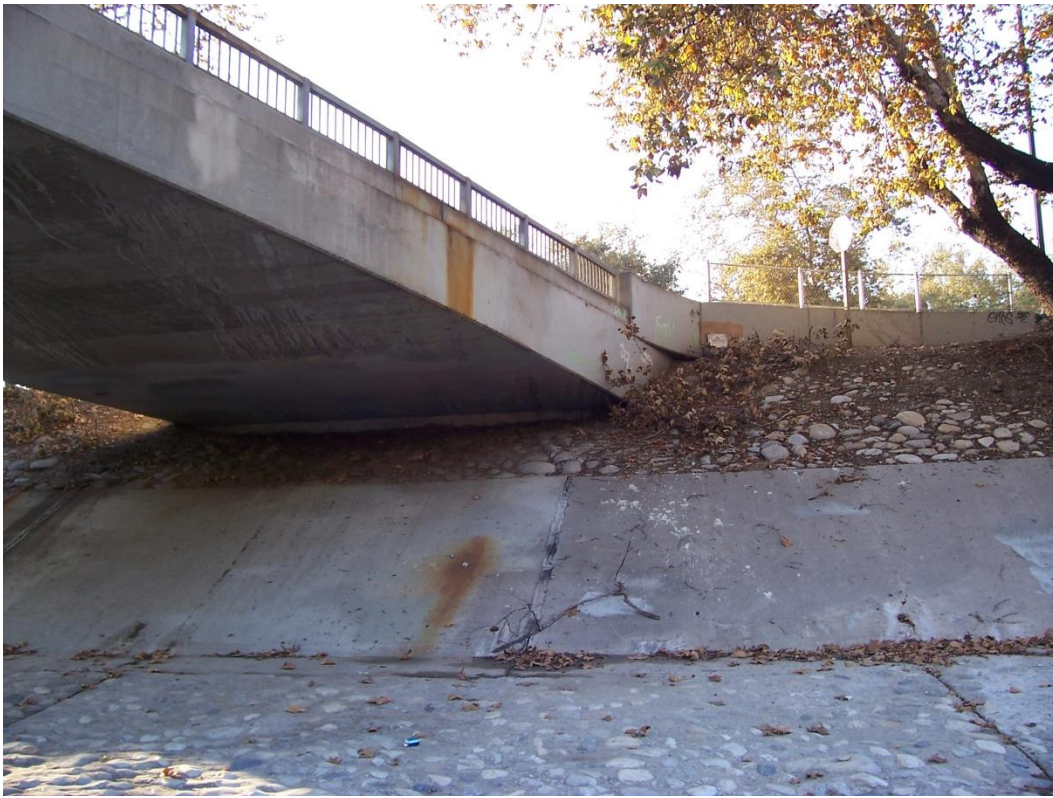
Section 1535 Downstream Right Bank Bridge Abutment
