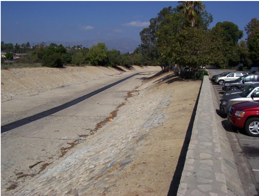
Section 2191.66 Looking Upstream
