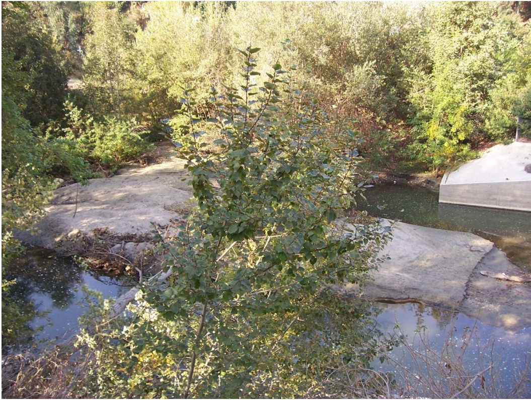
Section 2820 Looking Downstream Right Bank
