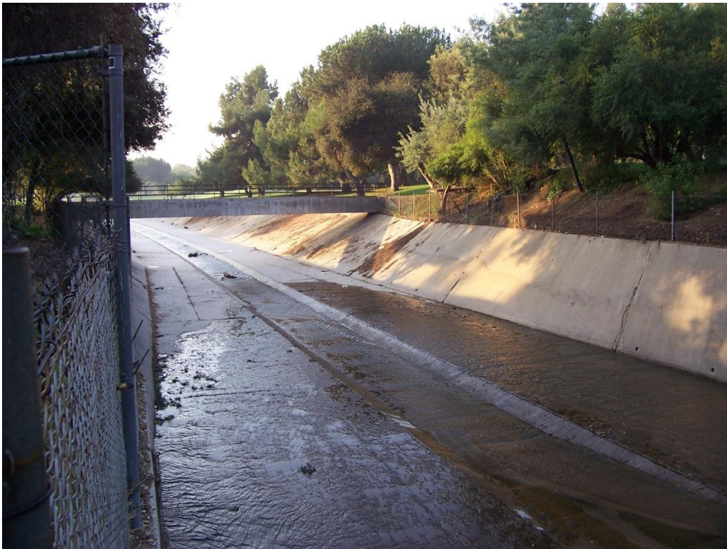
Section 3090 Looking Downstream
