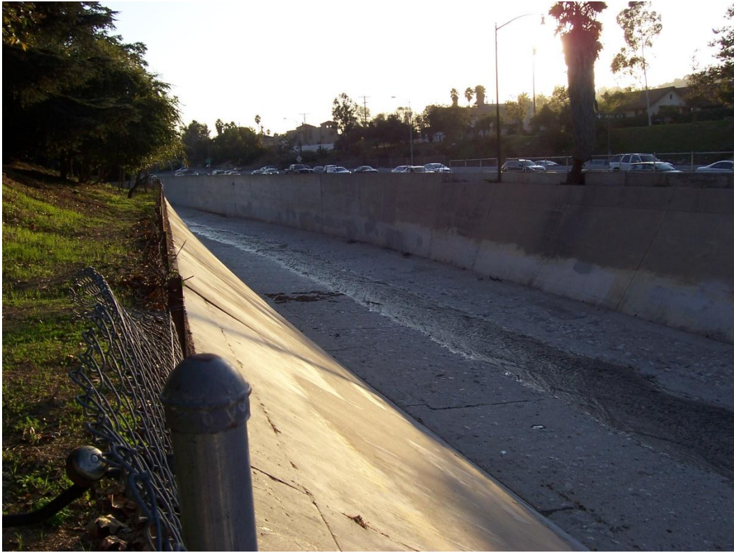
Section 598 Looking Downstream
