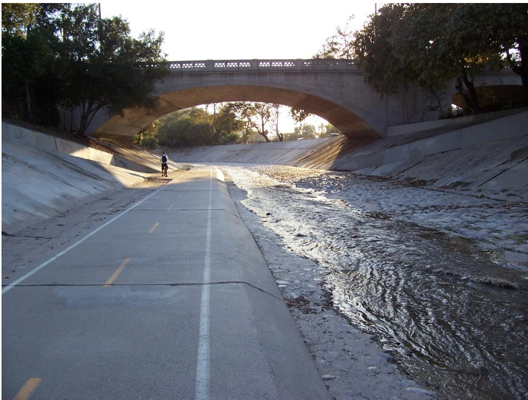
Section 1520 Looking Downstream
