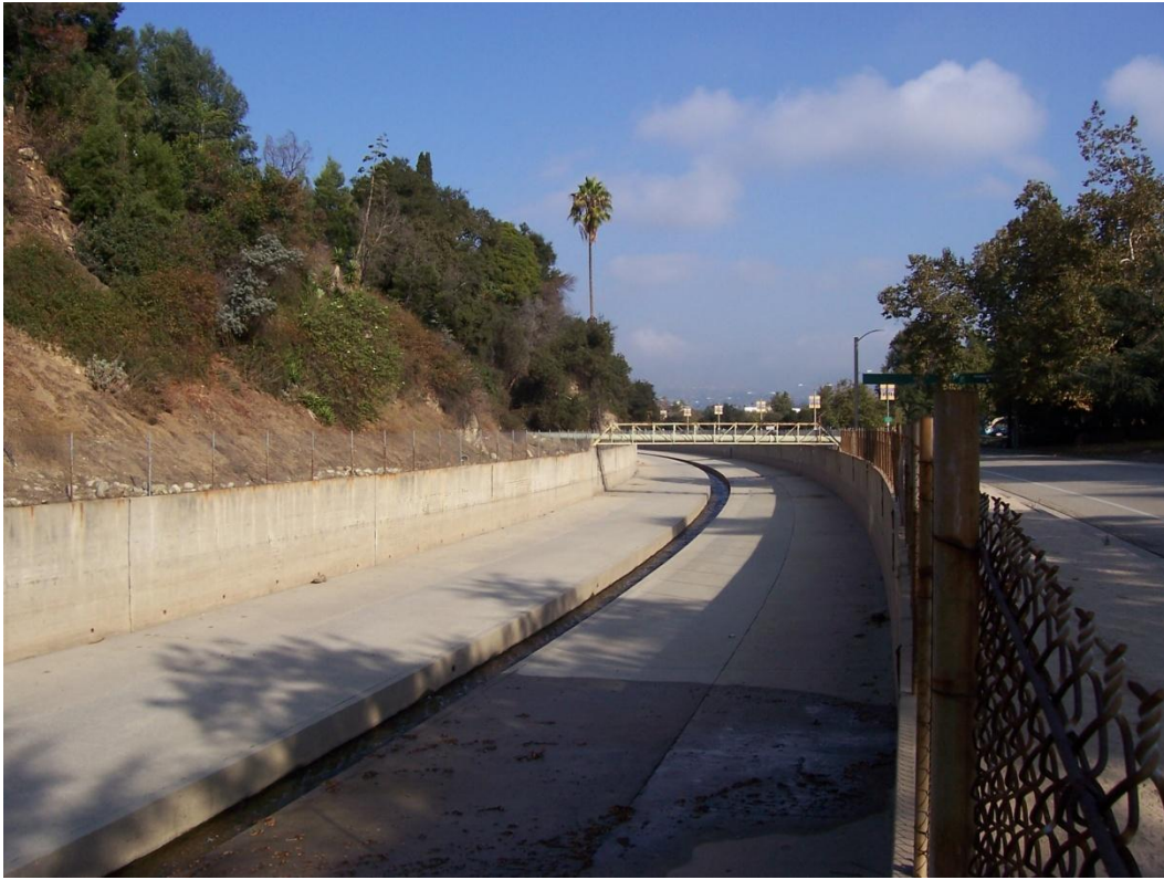
Section 2830 Looking Upstream
