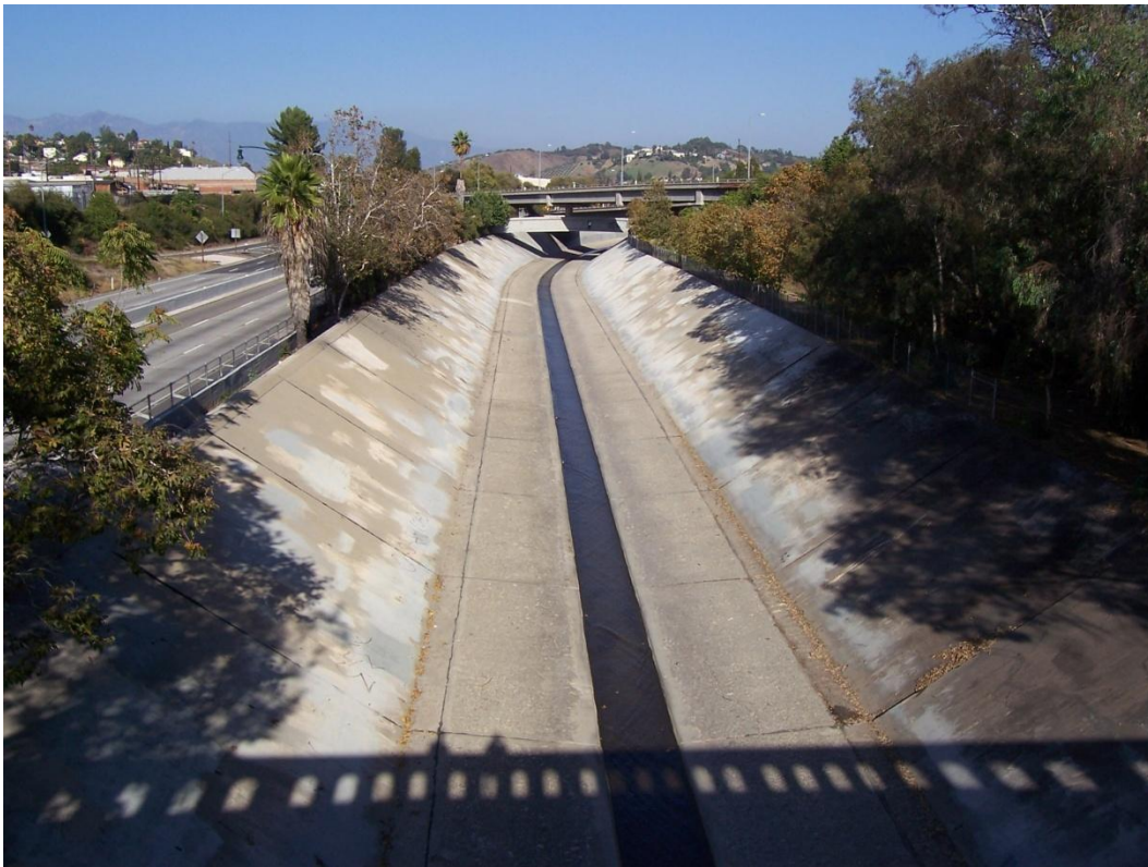
Section 180 Looking Upstream
