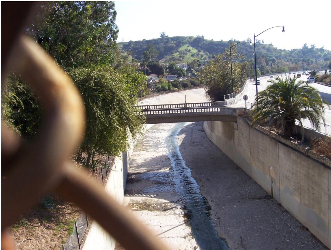
Section 508 Looking Downstream
