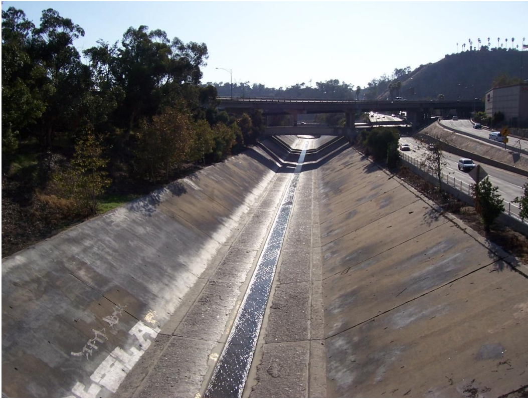
Section 180 Looking Downstream
