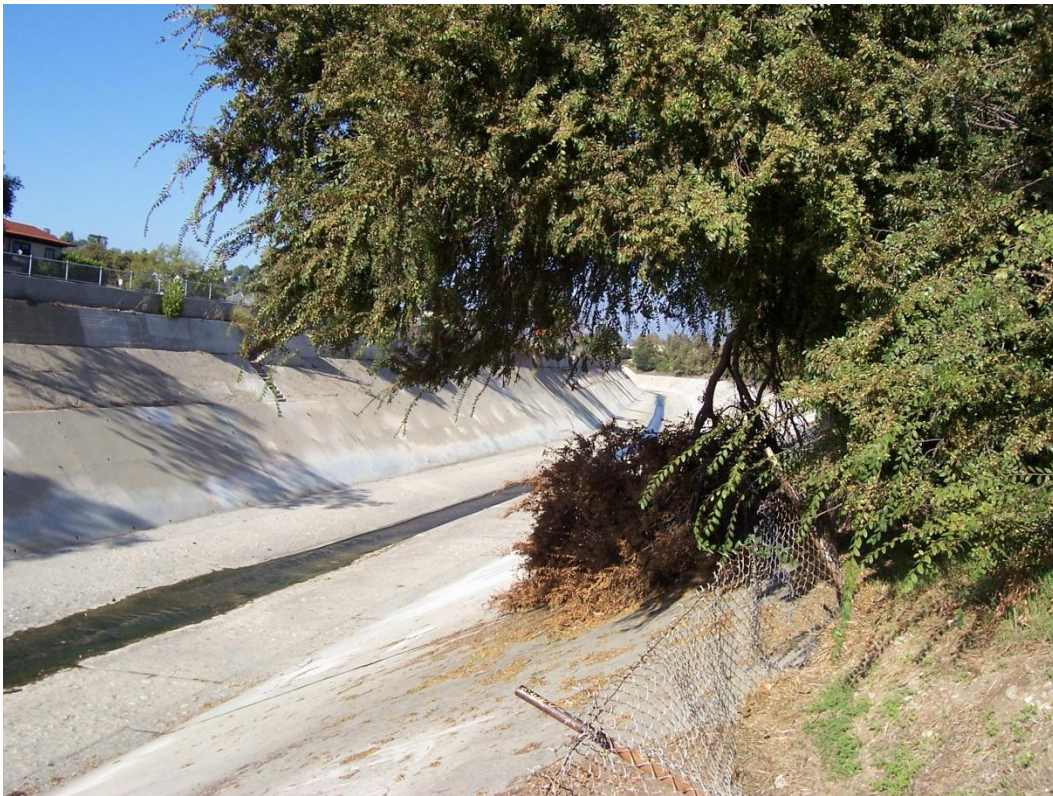
Section 376 Looking Upstream
