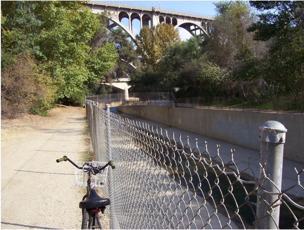
Section 2720 Looking Upstream
