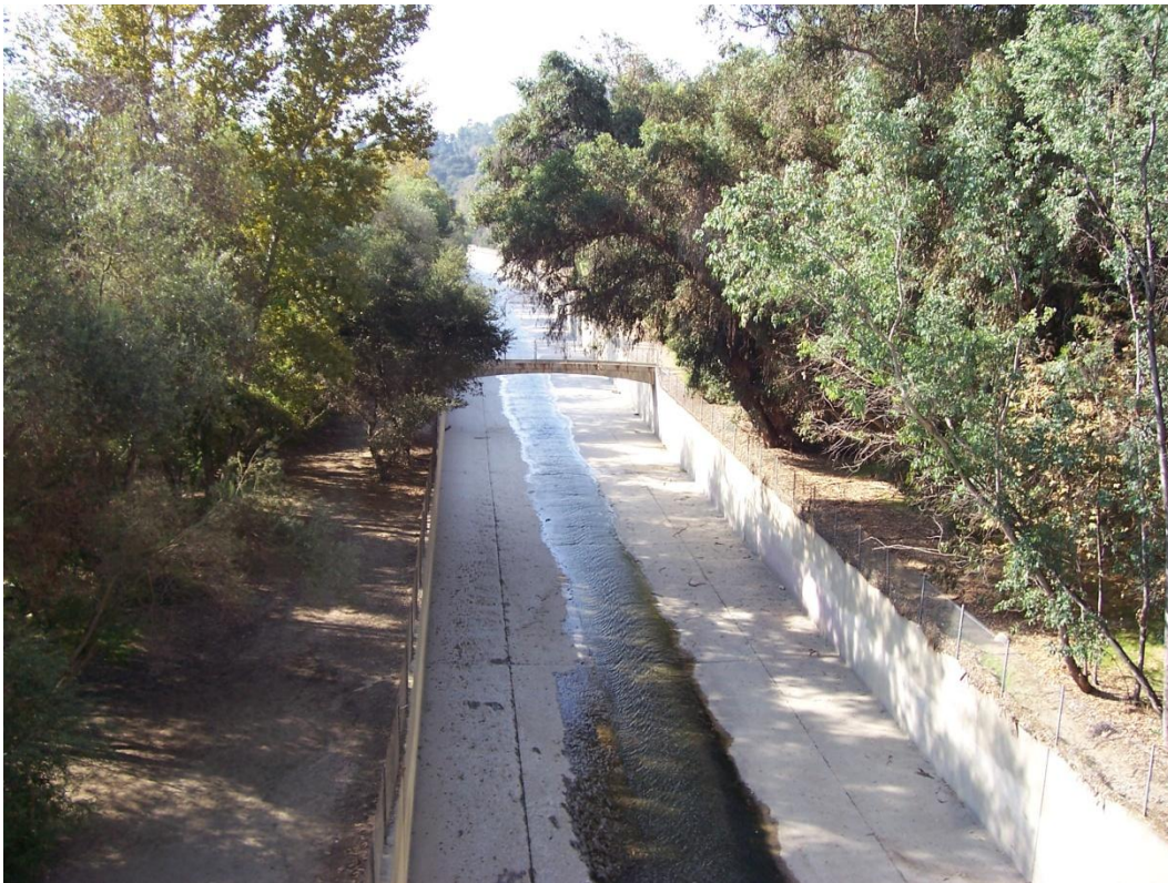
Section 2770 Looking Downstream of Entrance Structure to Channel
