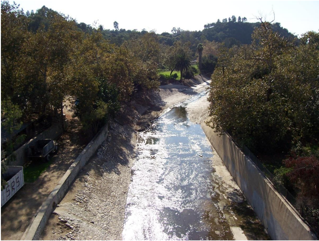
Section 1995 Looking Downstream
