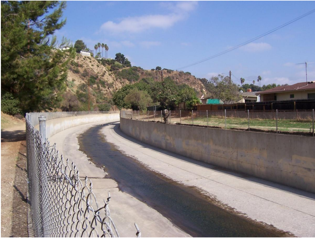
Section 2475 Looking Upstream
