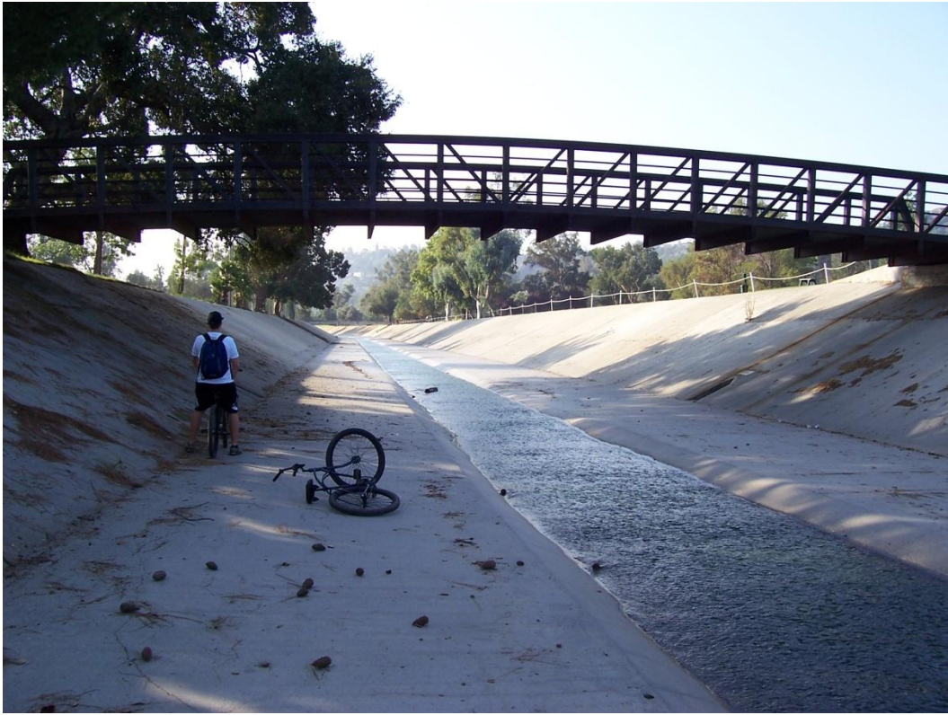
Section 3023 Looking Downstream
