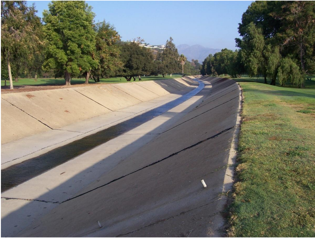
Section 3060 Looking Upstream
