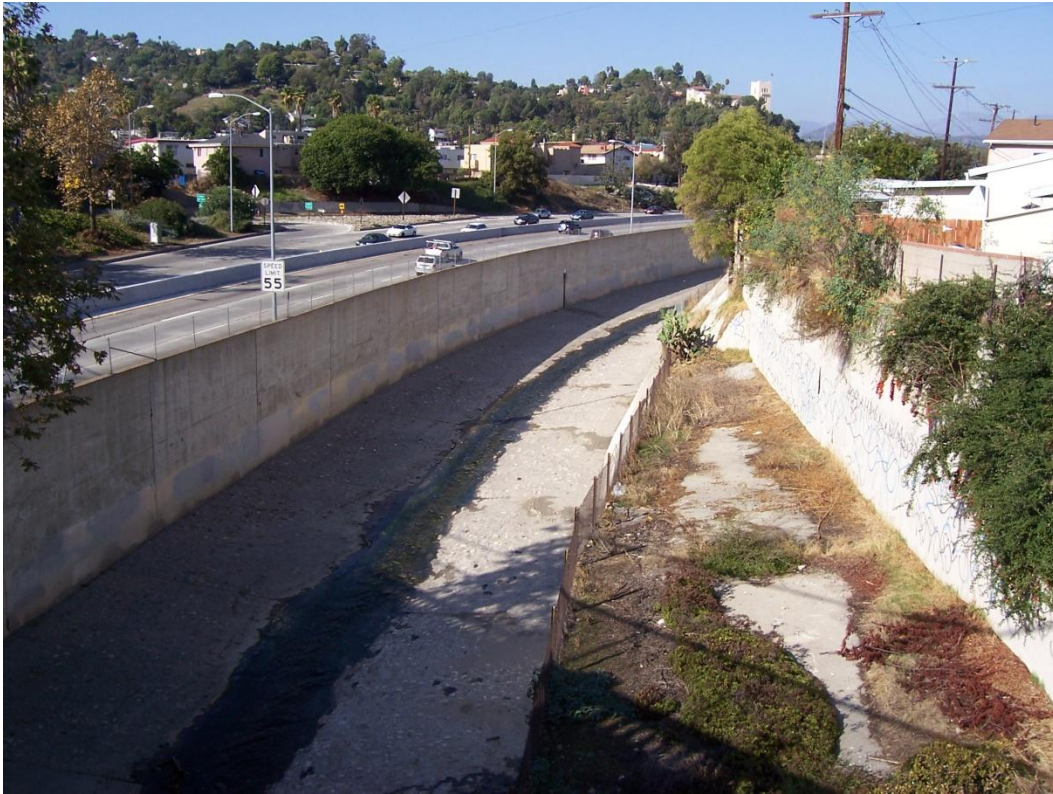
Section 508 Looking Upstream Left Bank
