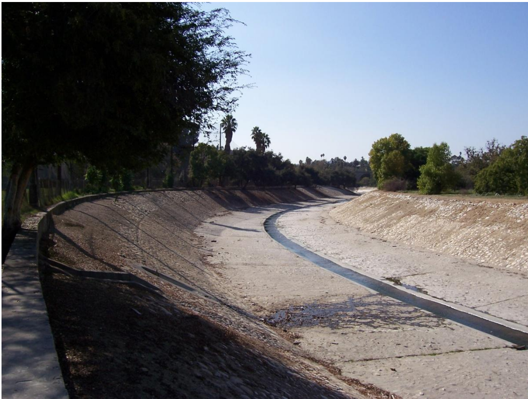
Section 2191.66 Looking Downstream
