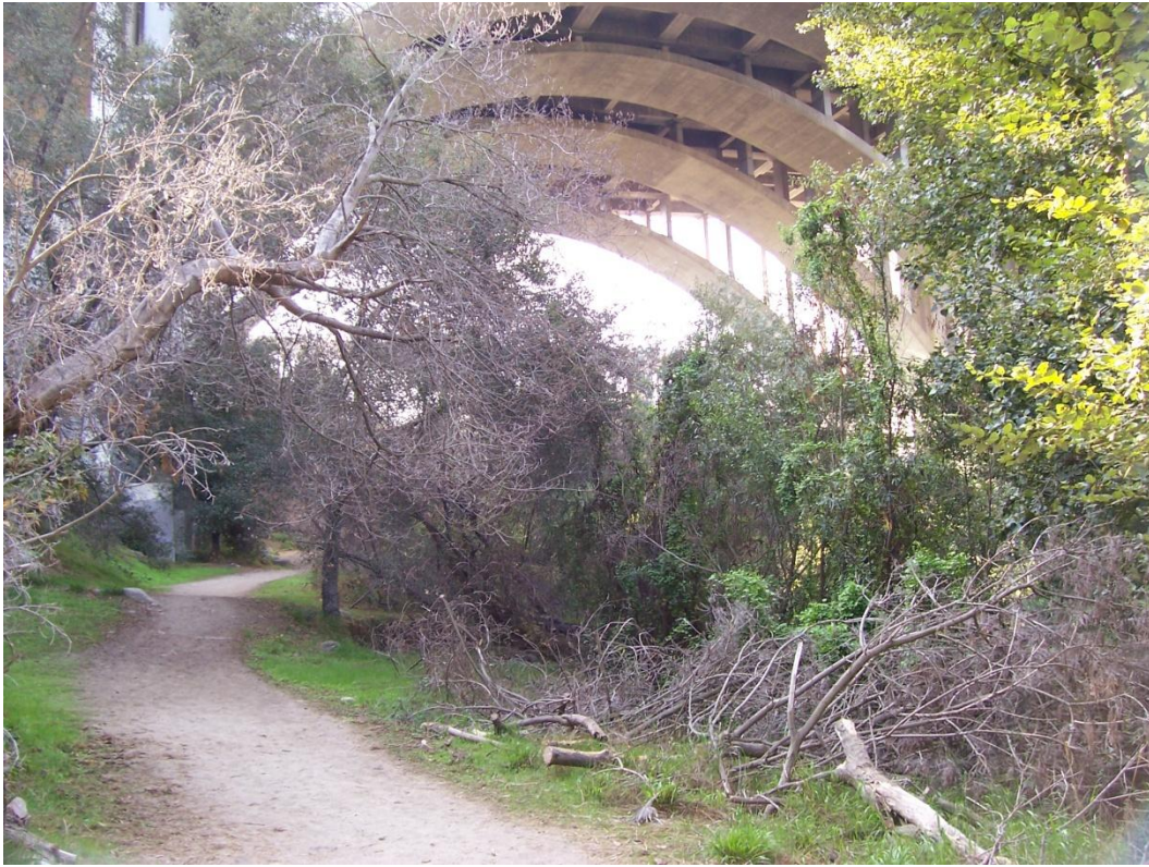
Section 2800+ Looking Downstream
