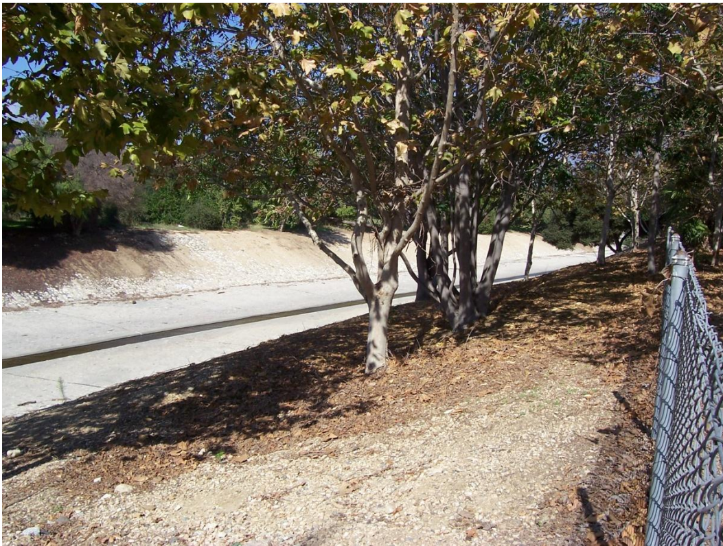
Section 2212.30 Looking Upstream
