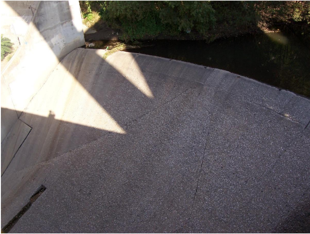
Section 2770 Looking Upstream Entrance Structure to Channel 3
