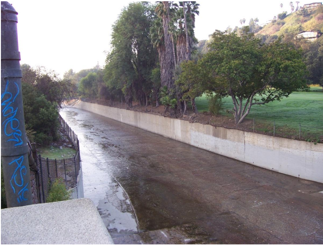
Section 3130 Looking Downstream
