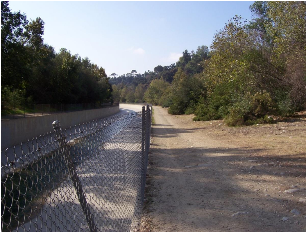
Section 2720 Looking Downstream
