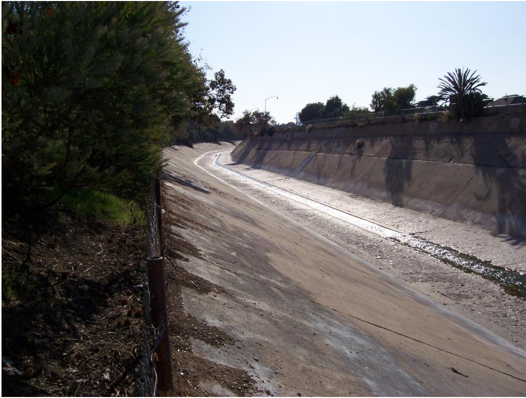
Section 405 Looking Downstream
