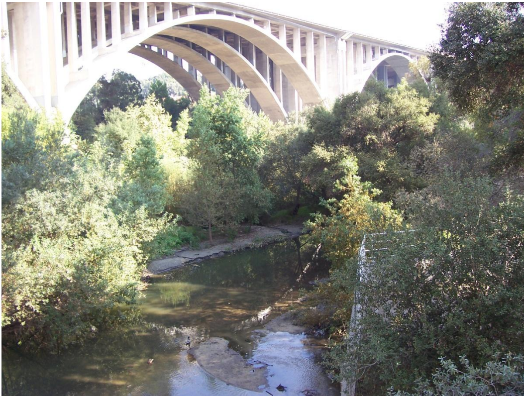
Section 2770 Looking Upstream of Entrance Structure to Channel 1
