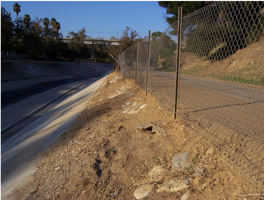
Section 1580 Looking Upstream Left Bank
