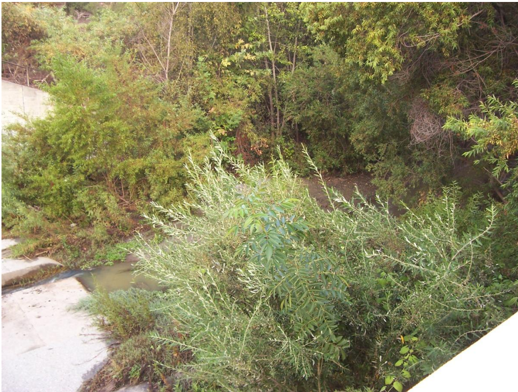
Section 3130 Looking Upstream
