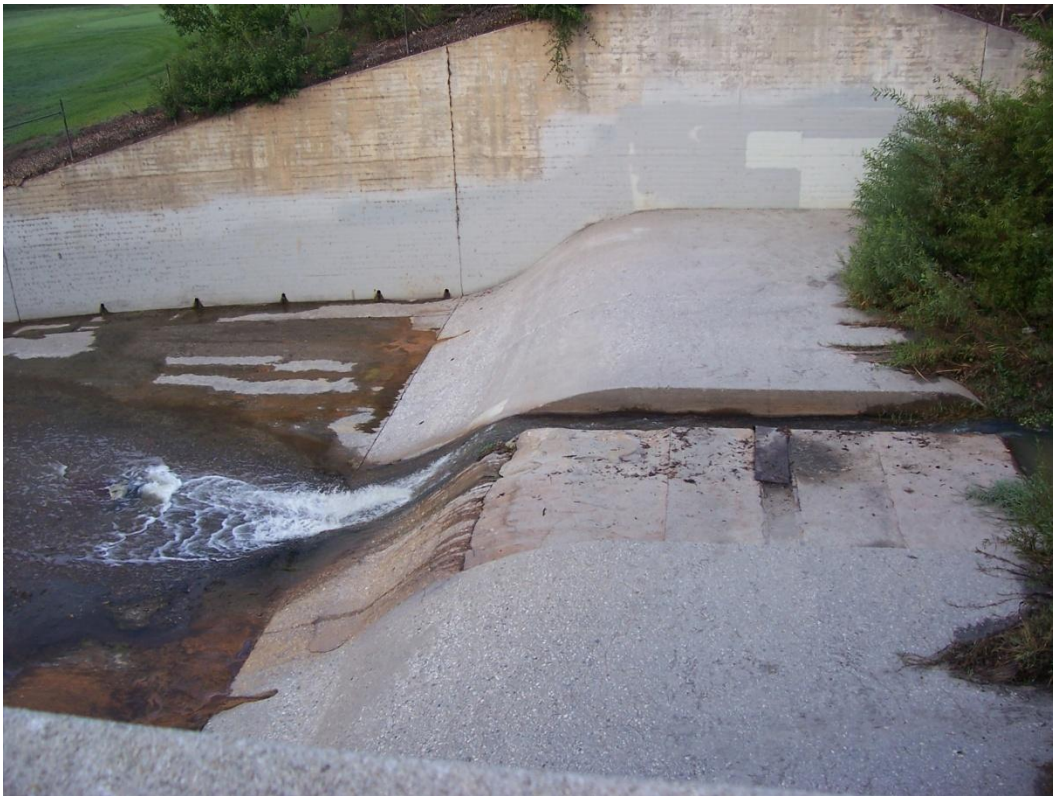
Section 3130 Grade Structure
