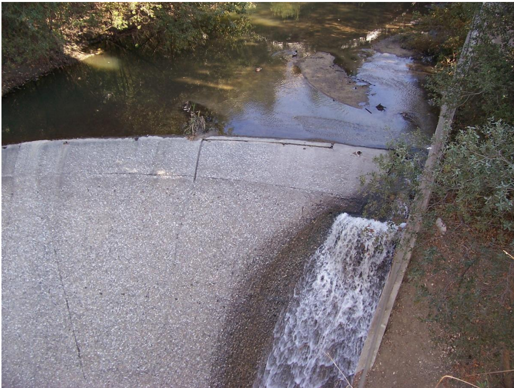
Section 2770 Looking Upstream Entrance Structure to Channel 2
