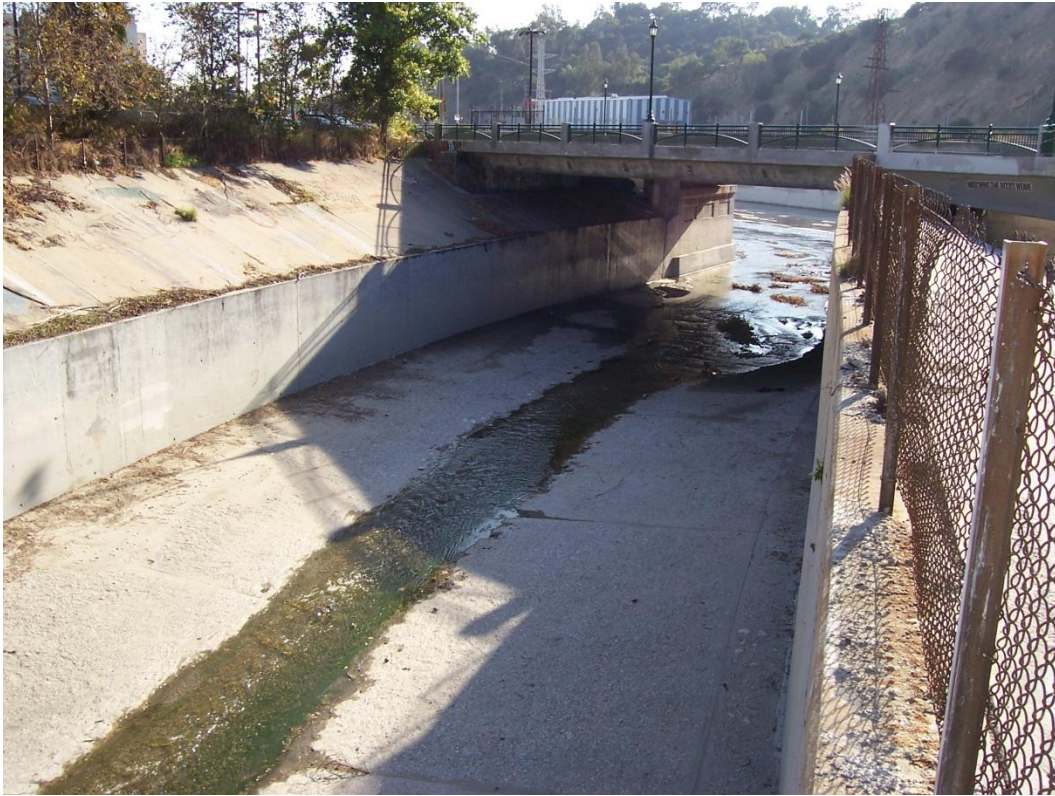
Section 10: Looking Downstream
