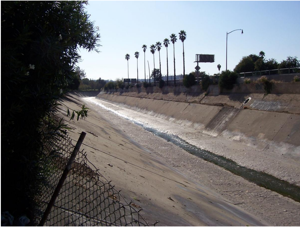
Section 376 Looking Downstream
