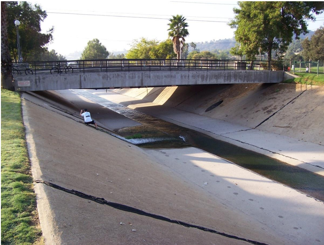
Section 3060 Looking Downstream
