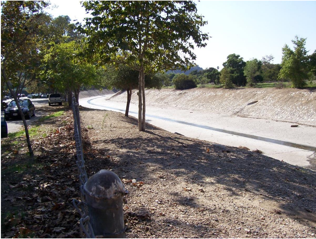
Section 2212.30 Looking Downstream
