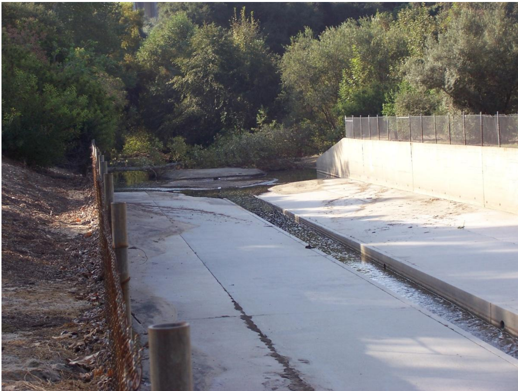
Section 2820 Looking Downstream
