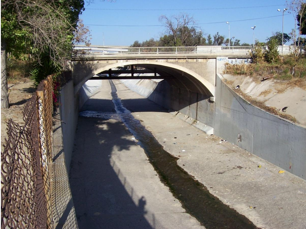
Section 10: Looking Upstream
